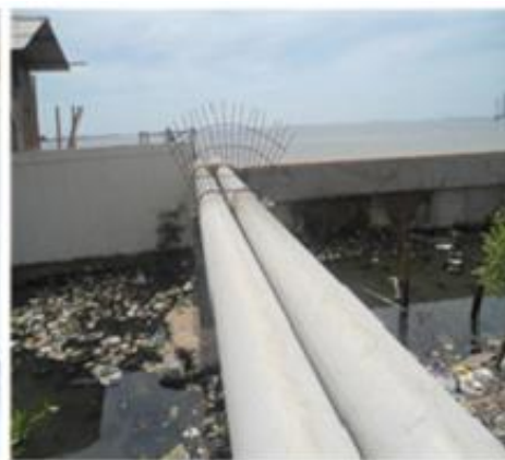
Two drainage pipes from station to Jakarta Bay
