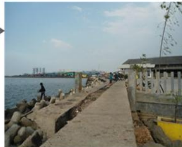
Break water to protect the port
