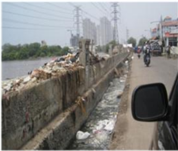
The dike to protect the settlement
