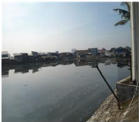
Waste water treatment pond (IPAL)
