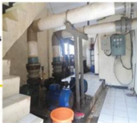
Four pumps in pumping station
