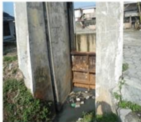
Sluice gate near the pumping station
