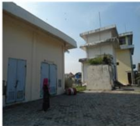
Pumping station at the edge of IPAL
