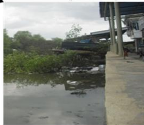
The dike of Asin River
