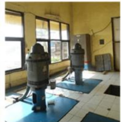
Four pumps in pumping station
